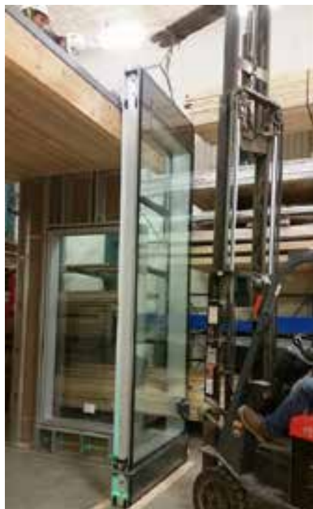
Worker installs a glazed curtain wall panel on a full-scale mockup of one of the corner bays of the 80 Atlantic project at the Carpenters' Union training facility in Vaughan, Ontario.
