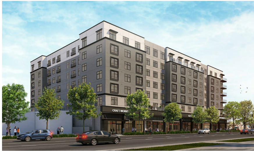
Anthem Properties Group is about to start construction on an eight-story apartment building on the 1500 block of S Street in downtown Sacramento, California. ANTHEM PROPERTIES GROUP
