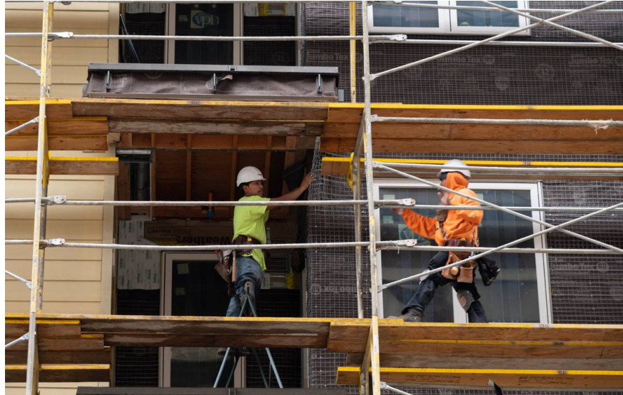
Building crews work at the Capitol Towers Tuesday in downtown Sacramento. The project replaces villas built in as part of a redevelopment project in the 1950s and '60s. Paul Kitagaki Jr. PKITAGAKI@SACBEE.COM
