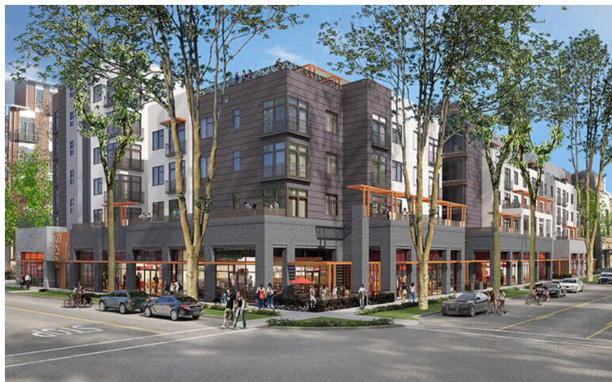
A new affordable housing apartment building is under construction at 1717 S St. in midtown Sacramento,
